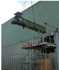
Demontage vorhandener Systeme Disassembly of existing systems
