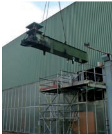
Demontage vorhandener Systeme Disassembly of existing systems
