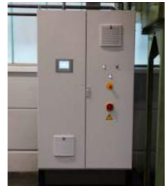
Installation der Steuerung Installation of the control system
