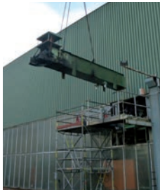
Demontage vorhandener Systeme Disassembly of existing systems
