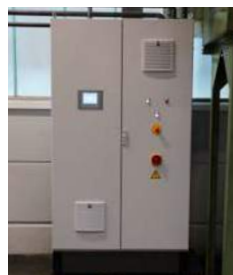
Installation et commande Installation of the control system
