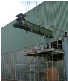
Demontage vorhandener Systeme Disassembly of existing systems
