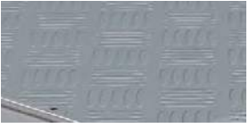
5 Structural metal plates to prevent slipping (on the largest box)
