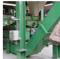
■ Scraper conveyor under a hopper system for aluminum chips
