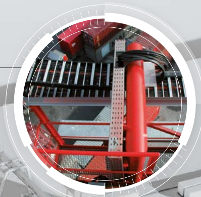
Rail Mounted Gantry (RMG)
